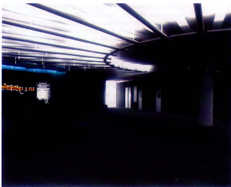
Figure 14. An indirect lighting system was designed to reduce glare on monitors in the London Underground control center.
